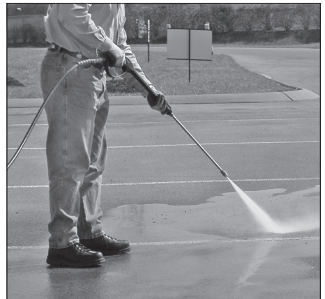
Figure 22 - Optimum angle to cleaning surface
